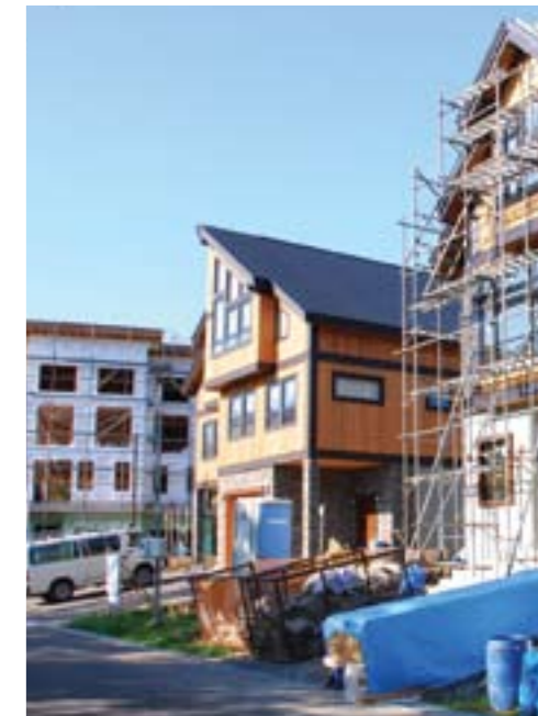
Buildings continue to go up in Niseko
