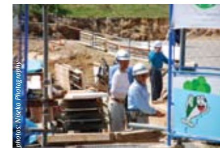
Laying the foundations
