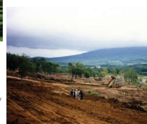
BEFORE... Photos of the prime patch of land ahead of construction
